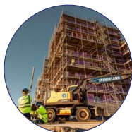
Sustainable new buildings
