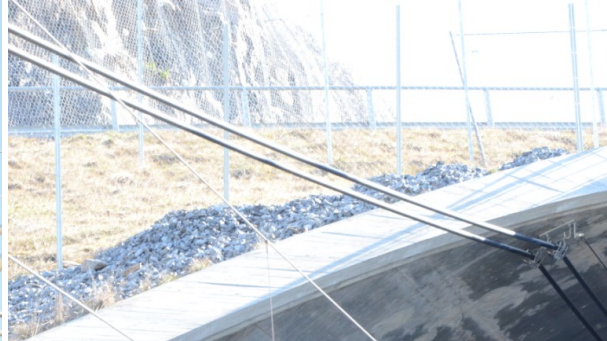
Figur 17.20 Kabel inn i tunnel
