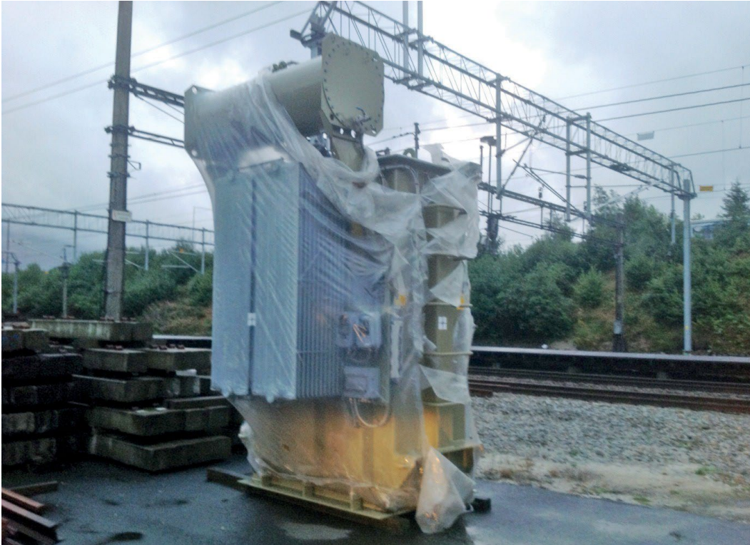
Figur 18.19 Autotransformator (AT)
