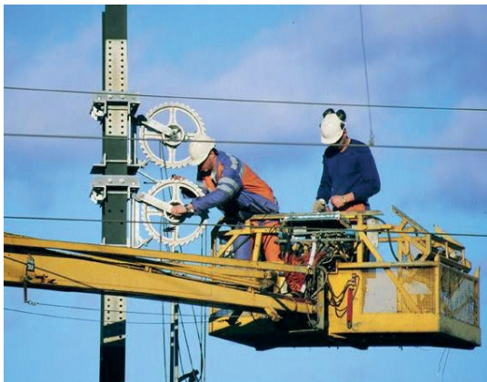
Figur 16.8 Loddhjul i tunnel
