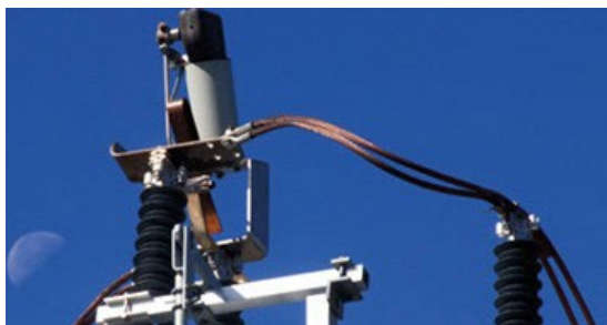
Figur 4.27 Lastskillebryter
